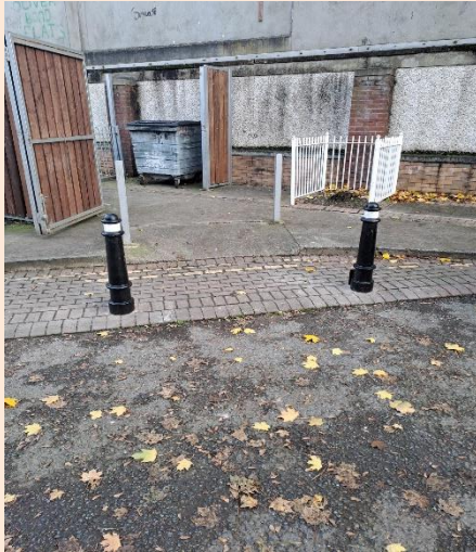
Oliver Bond: New poles have been installed to prevent parking in bin area at S & T blocks
